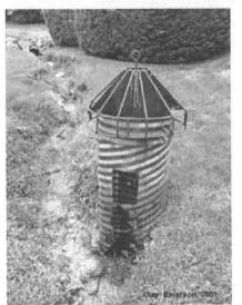
FIGURE 5-50 Rusted outlet structure. SOURCE: Reprinted, with permission, from Emerson. Copyright by Clay Emerson.
