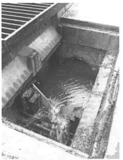
FIGURE 5-54 Weir flow used to measure flow rate. Courtesy of Robert Traver.
